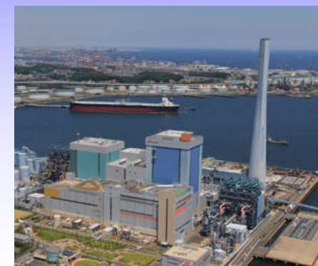
USC Plant in Japan
